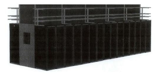
All computerized equipment generates heat. The Switch t-scif $^{TM}$  is designed to protect all of the customers in the facility from heat outputs. All equipment placed into the t-scif must vent the heat directly into the enclosed center aisle, where it is then contained and prevented from mixing back into the cold room.
