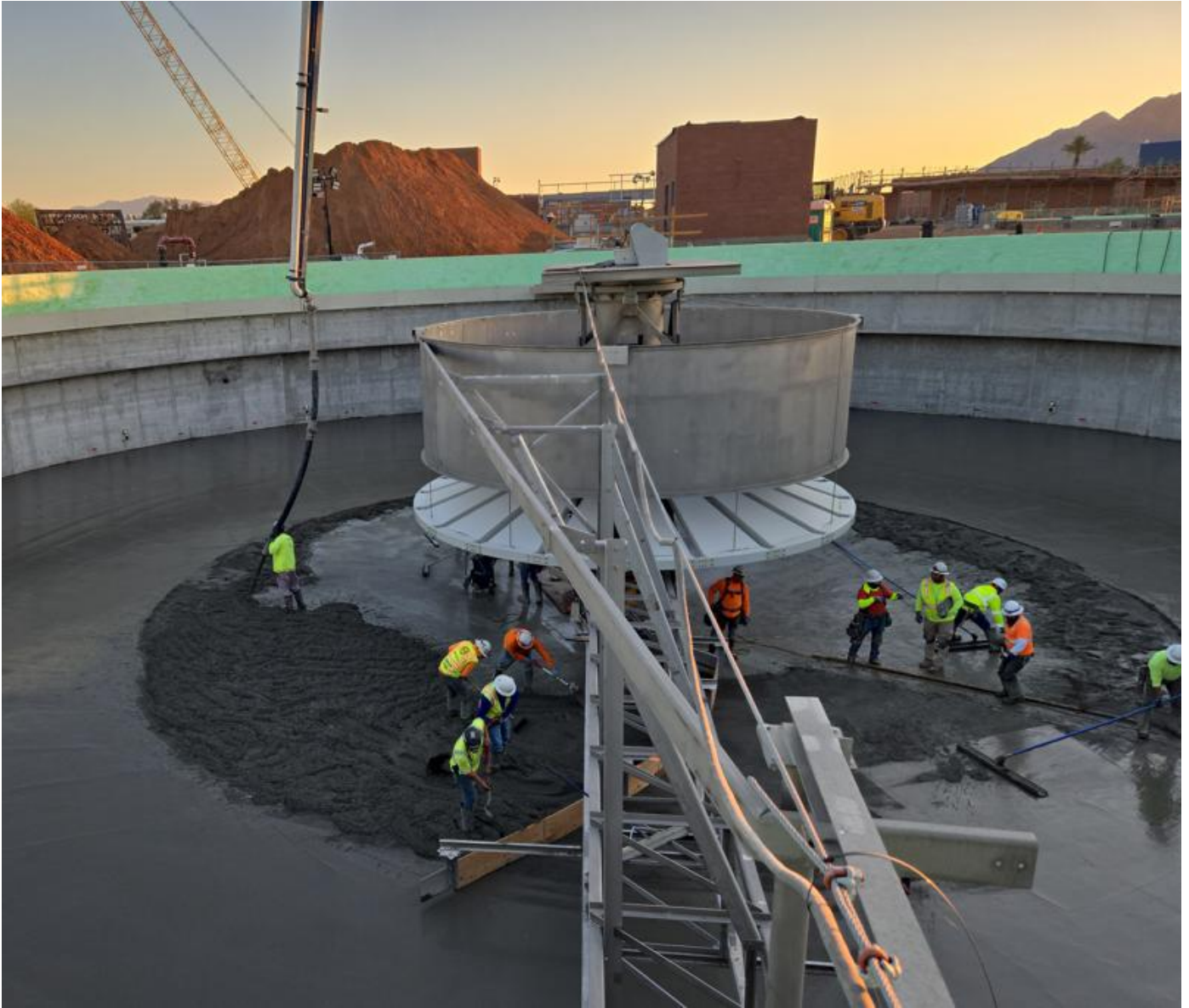
Placing a layer of grout at the primary clarifier hydraulic structure
