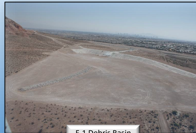
F-1 Debris Basin
