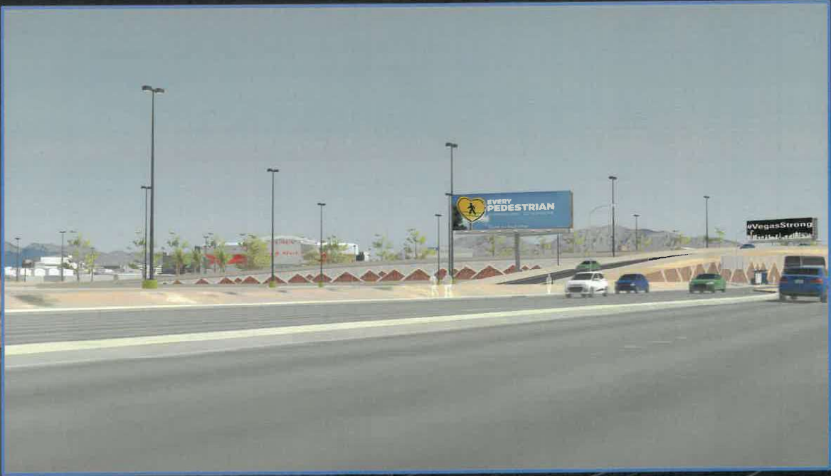
View of the Revised Shortened Overpass:
